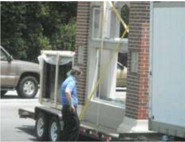
Installation day at last
