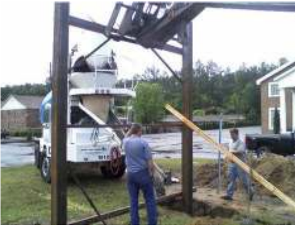
Setting the foundation posts
