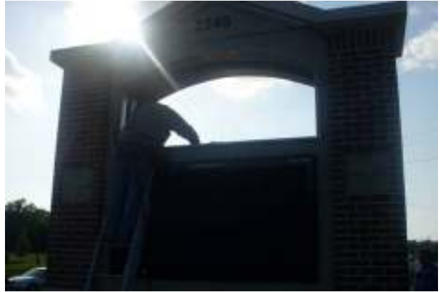
Installing the LED display panels
